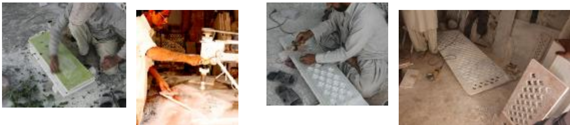
Figure 2.16. Manufacturing of Jali screens
