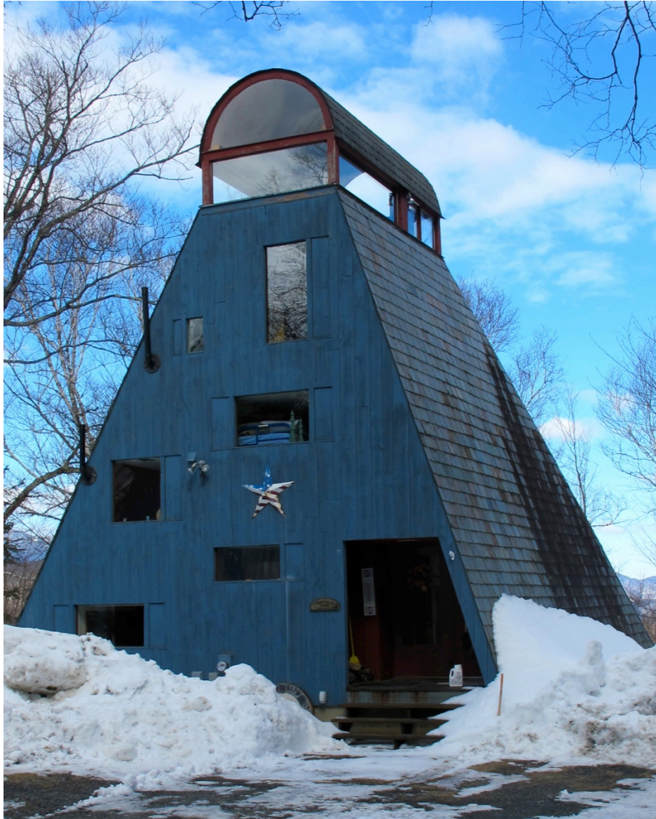
Fig. 9. Wadsworth House, constructed by David Sellers, Warren, Vermont, photo by author.
