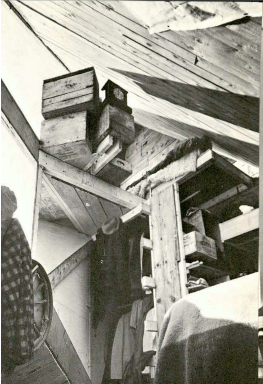
Fig. 2. Tack House Interior, 1965.
