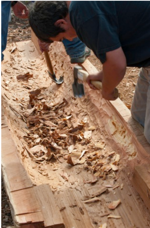
Figure 7: Digging Out by Team Ivy.
