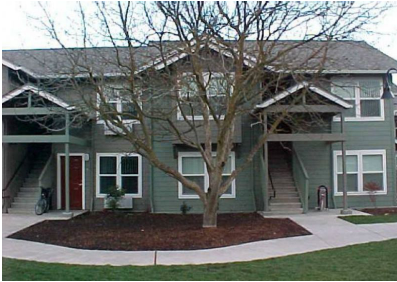
Figure 29: Lilac Meadow Apartments in Medford. Source: Housing Authority of Jackson County.
