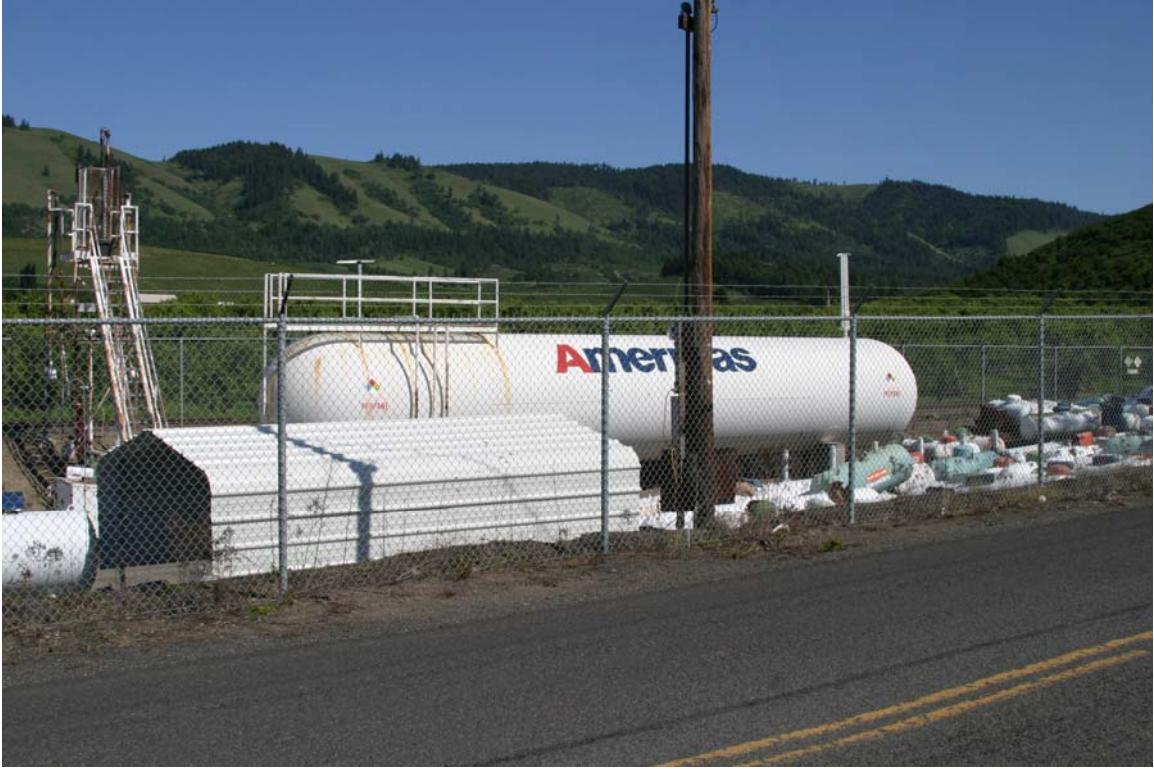
Figure 15: Propane Tanks in the Pine Grove District
