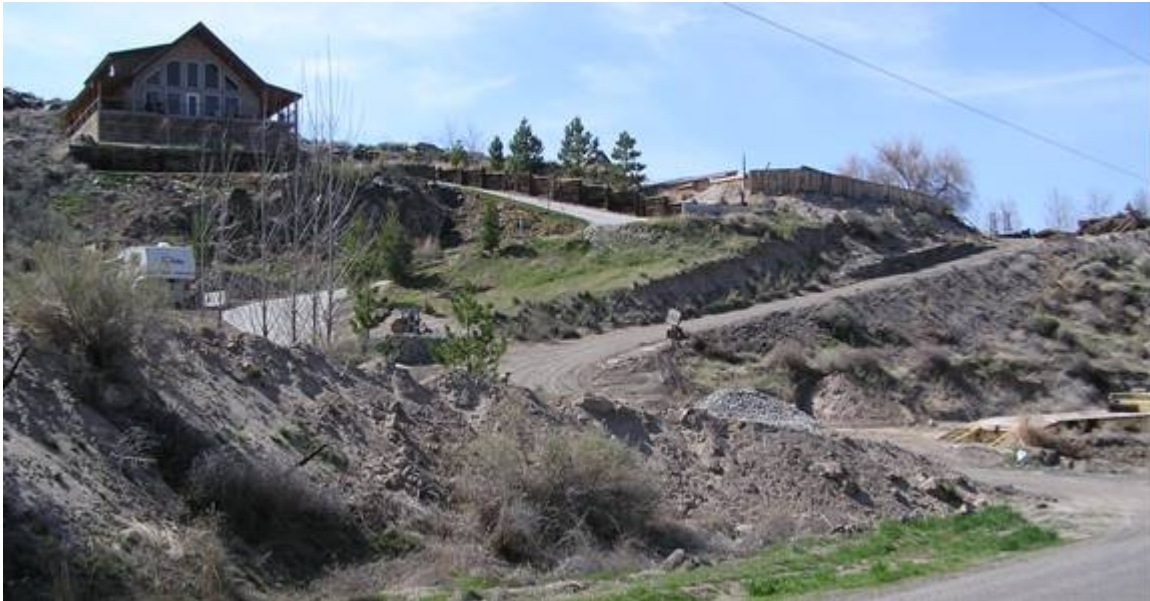
Figure 18. Bell Rapids Subdivision - Steep access road allowing passage only for a Command or wildland truck.
