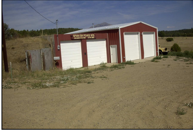
Gulnare Fire Station
