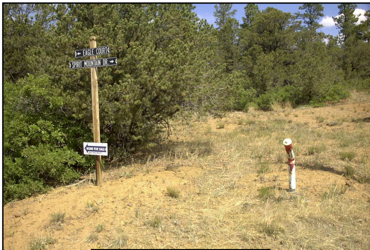
Fire Control Cistern
