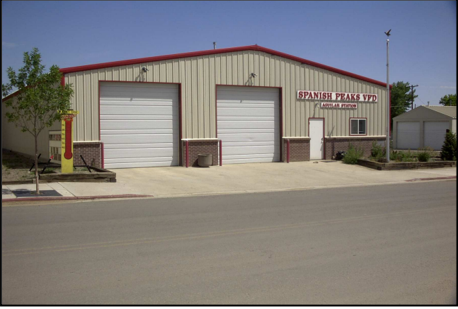
Augilar Fire Station
