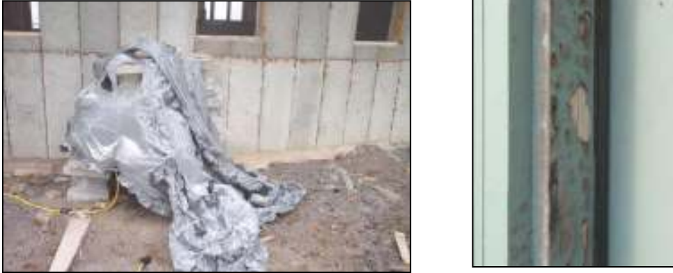
Figure 13. Affects of radiant heat 30 feet from flame
