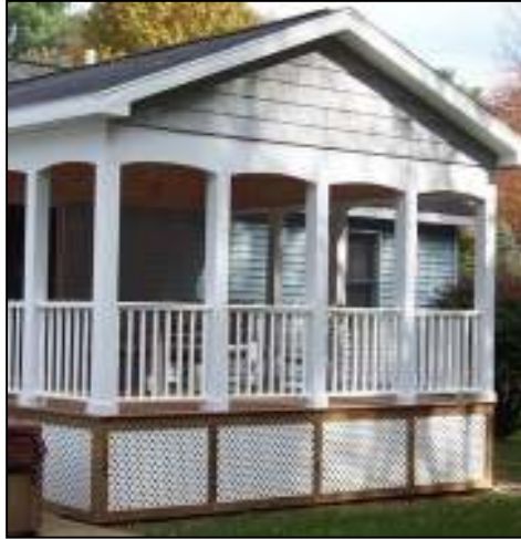
Figure 29. Screened decks restrict access from windblown debris
