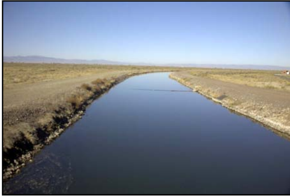
Bureau of Reclamation Closed Basin Canal
