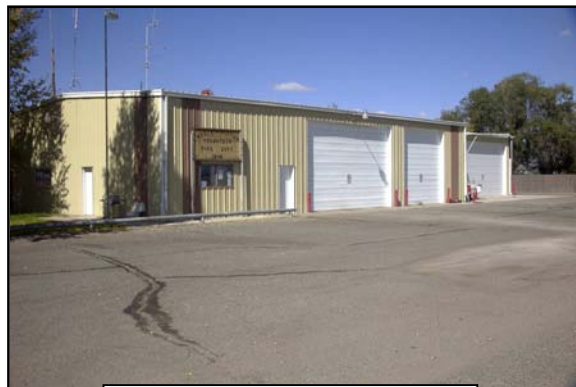
Hooper Fire Station
