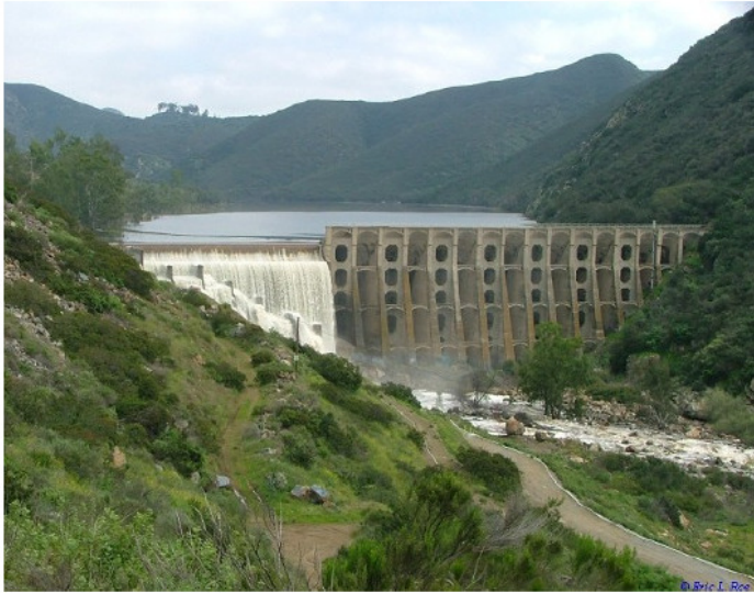
Lake Hodges Dam
