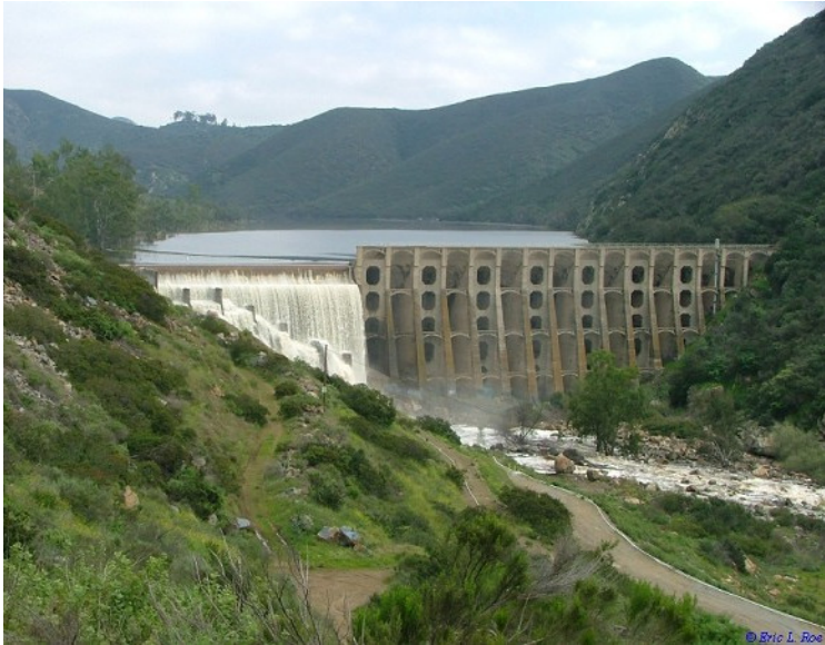
Lake Hodges Dam
