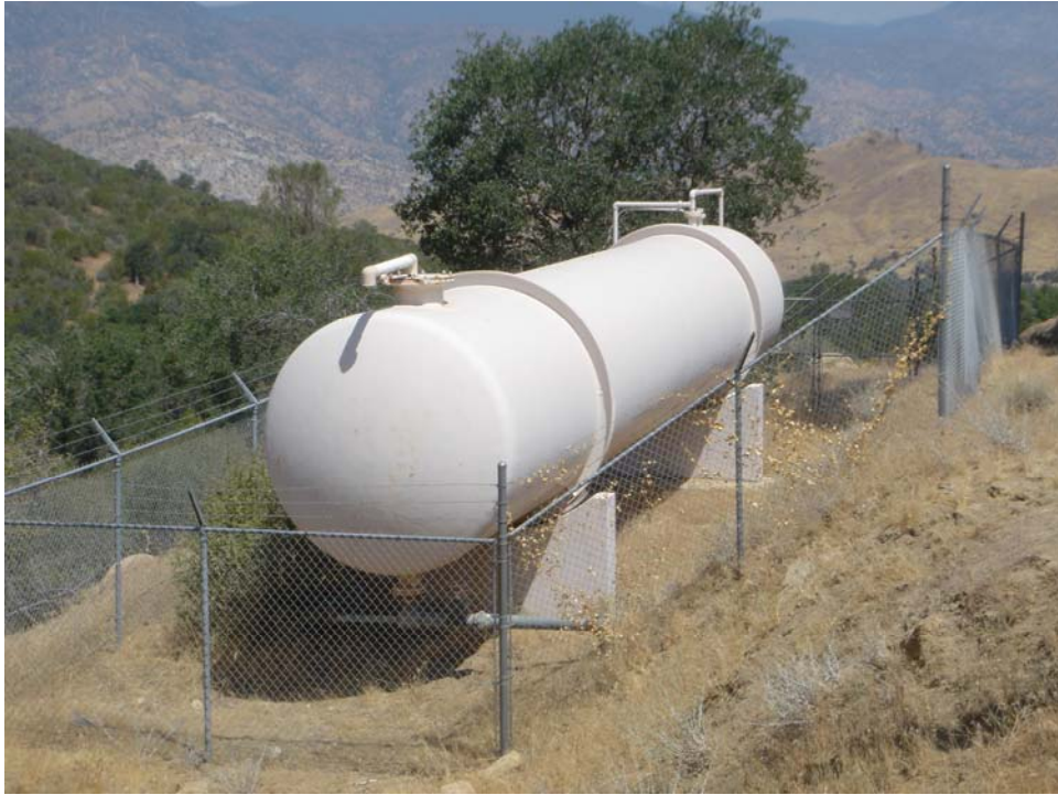
9000 gallon water tank located just north of 974 South Alpine
