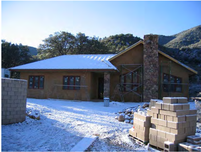
Photo E.2. Firewise home construction
