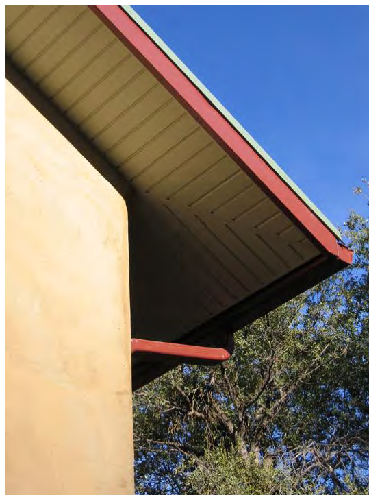
Photo E.3. Firewise rooftop and soffit
