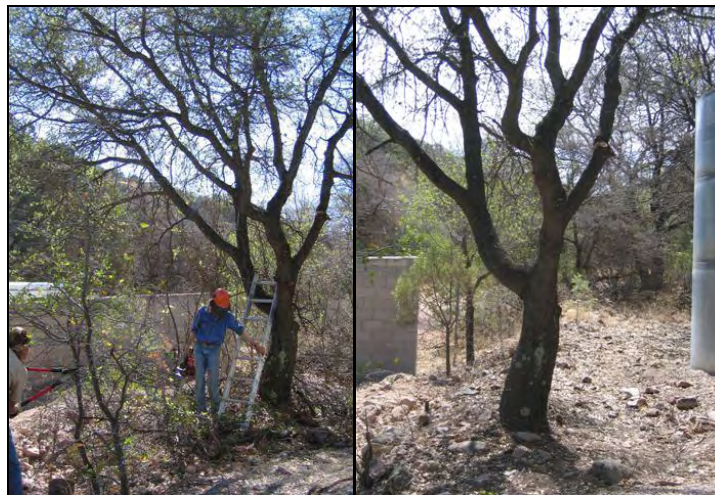
Photo 4.1. Before- and after-construction pictures of a home ignition zone firebreak
