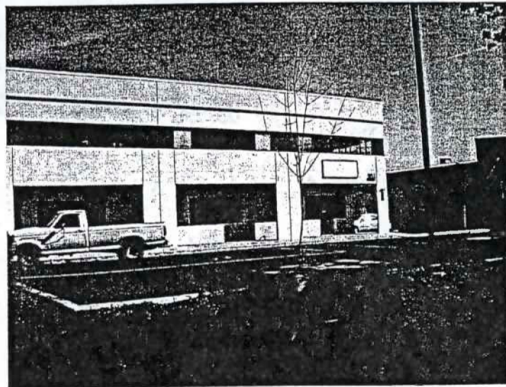
Existing business park on property located east of TL 400
