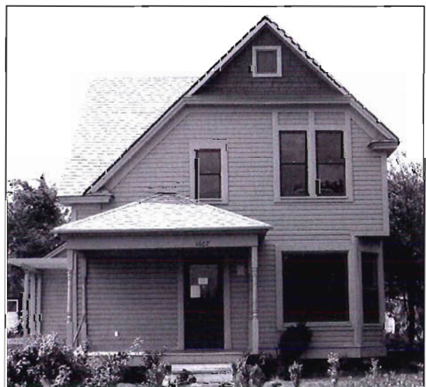
The historic character and street appeal are restored after rehabilitation of the siding, reconstruction of the trim and repainting
