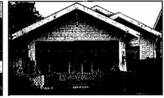
Bungalows generally have low to moderately pitched gable roofs supported by brackets.
