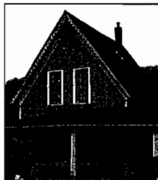
Gothic style influences. Steeply pitched gable roof with decorative fascia
