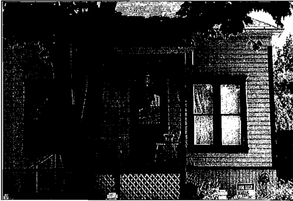
Original window and door types common in the District: paired, 1/1, double-hung wood sash windows
