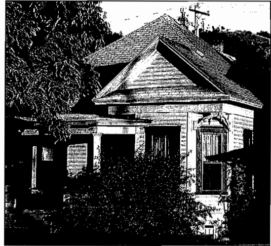
One of the many small Queen Anne cottages in the Mill-Pine neighborhood that retains architectural integrity and enhances the neighborhood
