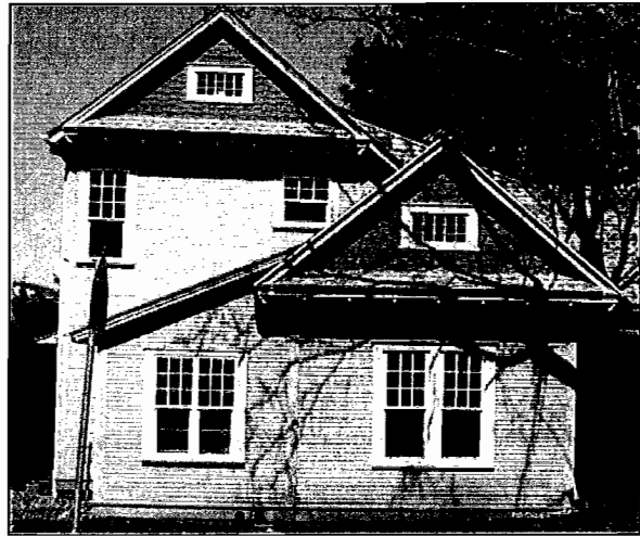
Height and Scale: The addition (left) on the Queen Anne cottage is too high and out of scale with the house. Although consideration was given to applying compatible design elements, the original house becomes “lost”
