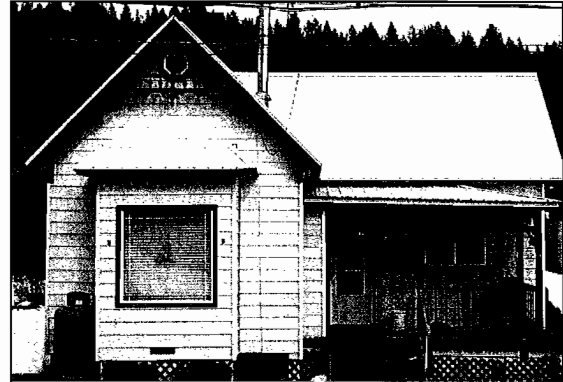
Vernacular Queen Anne cottage with incompatible new picture window and aluminum slider
