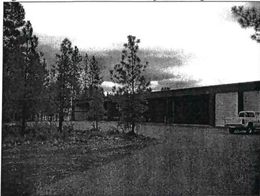
Figure 8: Public Works Facilities Adjacent to Figure 7
