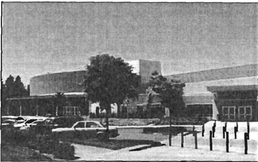
The entrance to Lakeridge High School presents a modern façade of concrete and glass.
