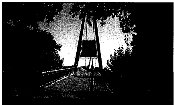
Bicycle/pedestrian suspension bridge in Frankfurt, Germany
