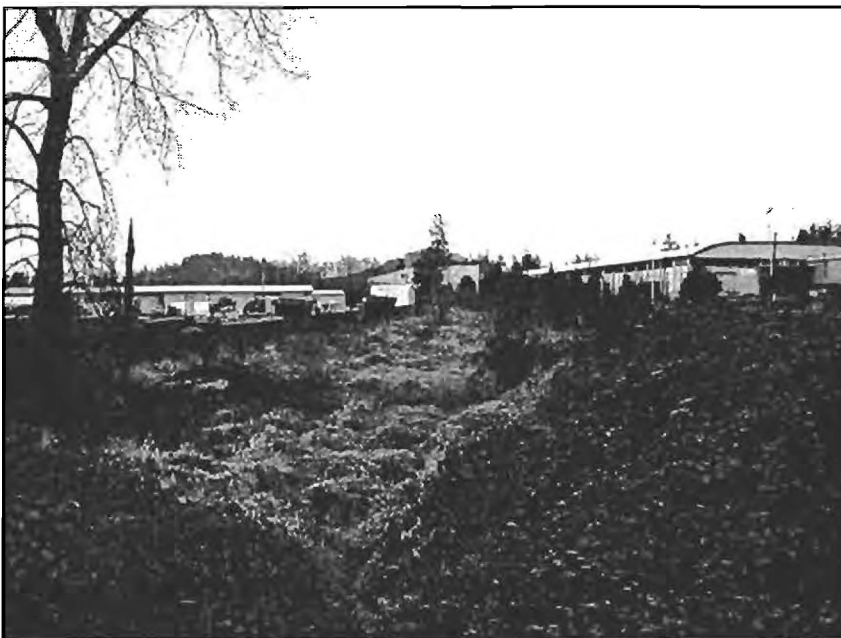
RGS-6 facing east taken from the west end
