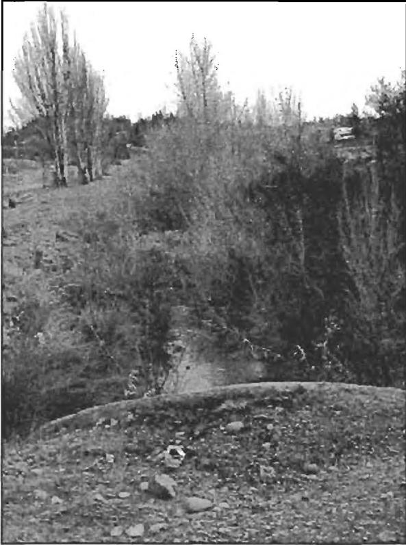
RGS-2A facing south at fish culvert
