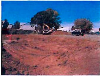
Above: Excavating the soil
