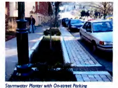
Stormwater Planter with On-street Parking
