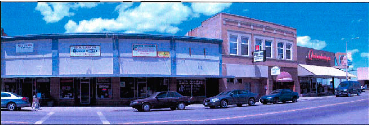
Existing sidewalk widths and deep awnings make tree planting in some parts of downtown difficult
