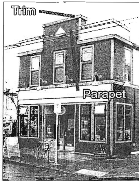
Figure 10A-57-210i. Parapet on a Flat Roof
