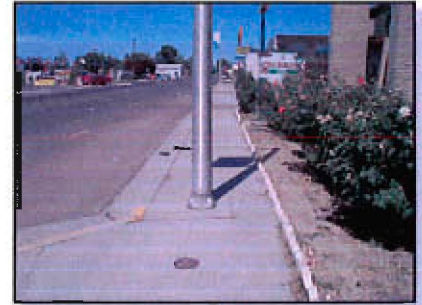
This light pole reduces the passable sidewalk width on SW 1st Street near SW 1st Avenue
