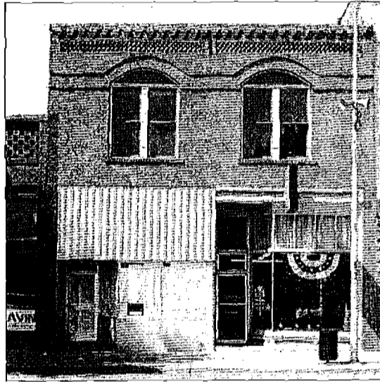
This building exhibits an original storefront on right with alterations occurring at the left.
