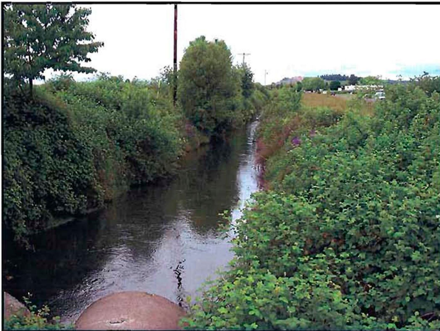
Irrigation Channel near Industrial Way
