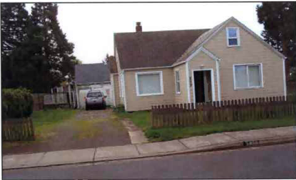
Existing dwelling fronting West M Street
