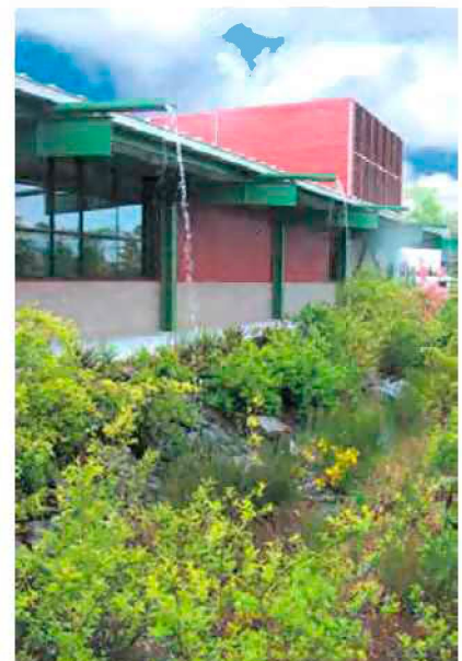
Capturing stormwater run-off from buildings in landscaped swales
