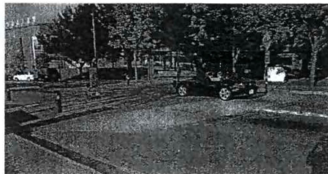
Raised intersections and changes in materials at gateways can improve pedestrian crossing safety and reduce traffic speeds.
