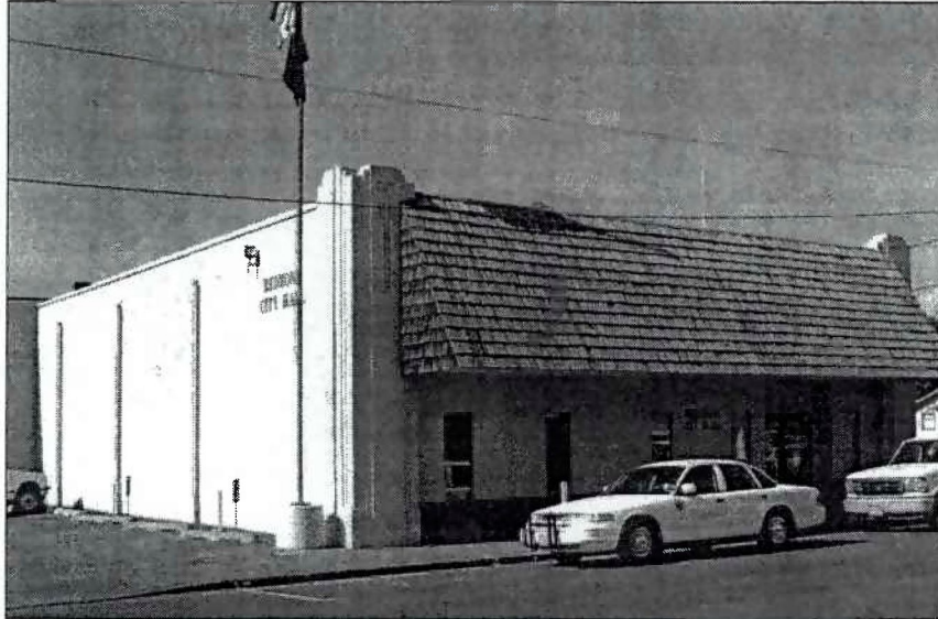
City Hall before Shake Awning was Removed
