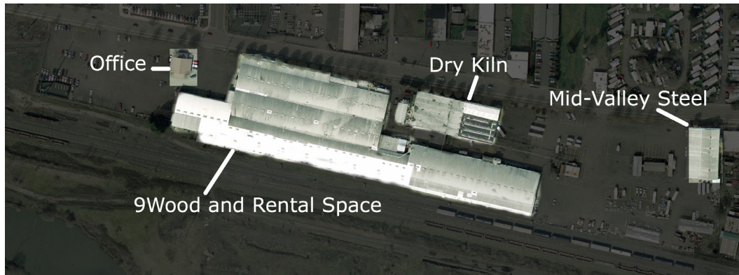
Figure 10: Existing structures on the Nicolai property.(Ludington 2013).
