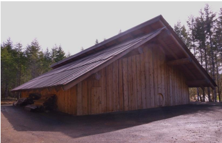
Figure 6. Main façade of the Achfa-hammi Plankhouse. View looking east ( photo by author ).
