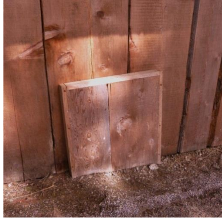
Figure 9. Wood panel designed to cover concrete pier for wood support beam (photo by author).
