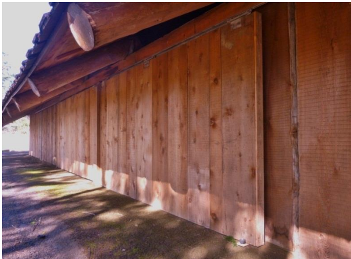
Figure 14. Sliding wood doors on south elevation. Note metal sliding track near the top ( photo by author ).
