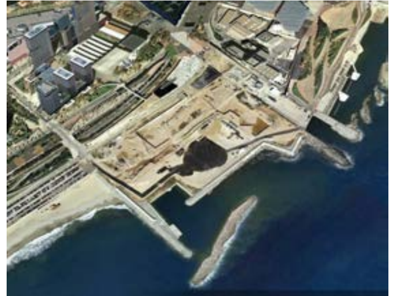
Existing Site Conditions Source - Google Maps
