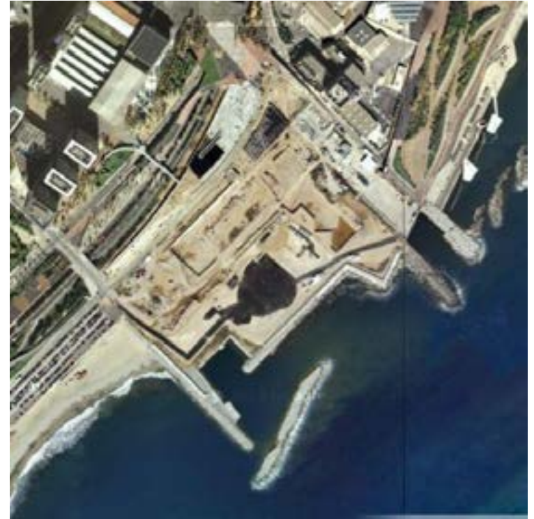
Existing Site Conditions Source - Google Maps
