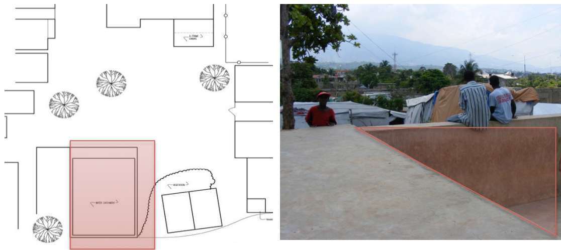
Figure 5.28. Location of a large water cistern in Save the Children, highlighted in red. It was empty at the time due to a dry spout of weather.
