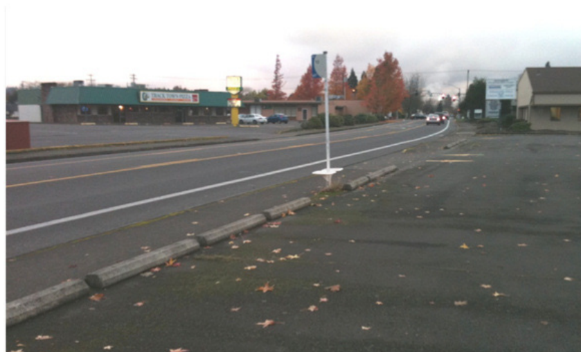
Figure 36: Centennial Boulevard – before.
