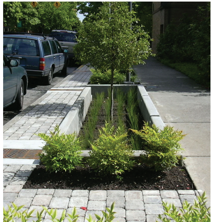
Figure 57: Bioswale in Atlanta.
