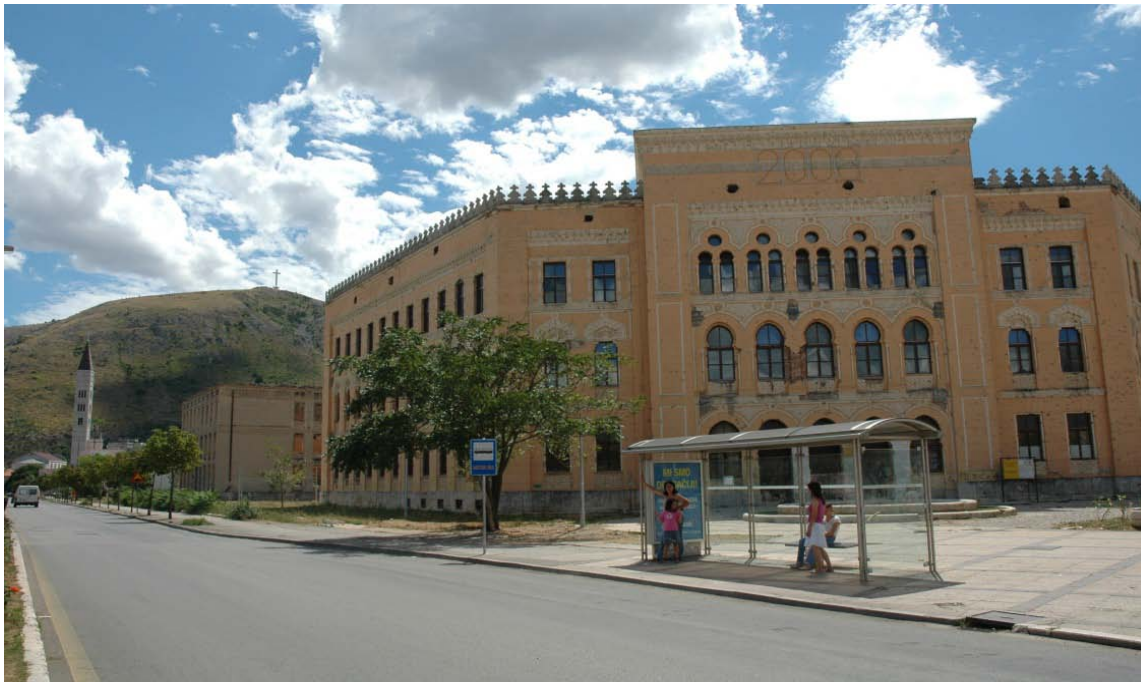
Figure 8. The Old Gymnasium. (author’s photograph 2006).
