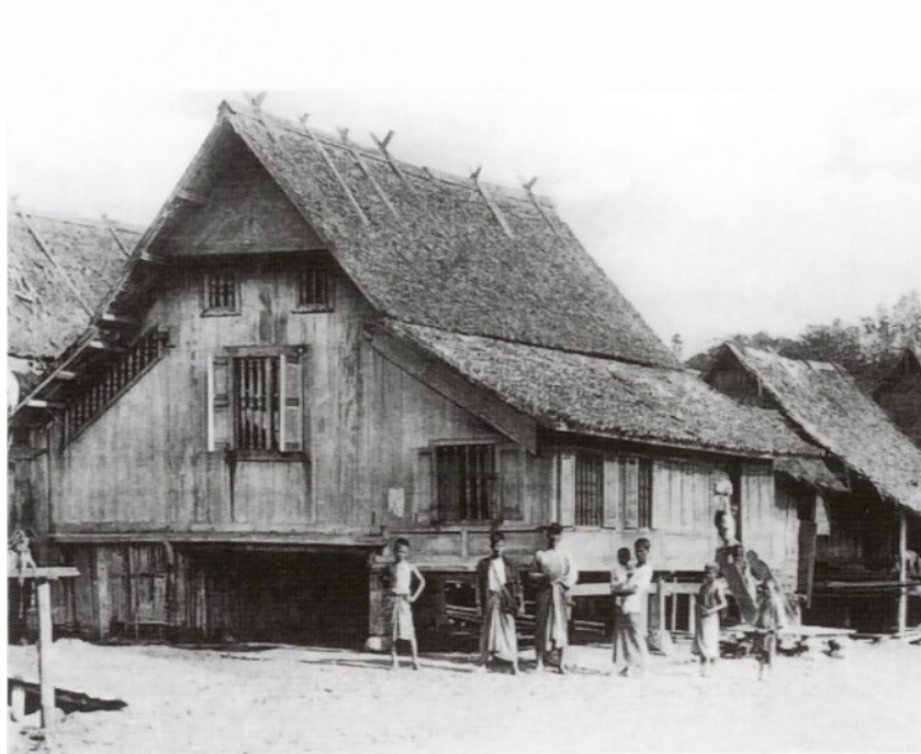
Fig. 2: Traditional Malay Home, Singapore (Davidson, Julian. Black and White: The Singapore House 1898-1941 . Talisman Publishing, 2006: 14)
