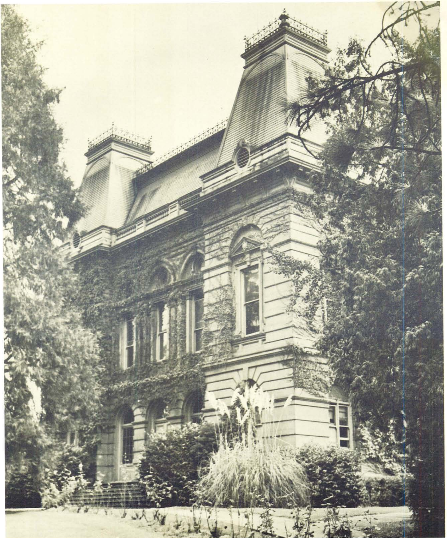
Villard — men's dorm and classrooms
