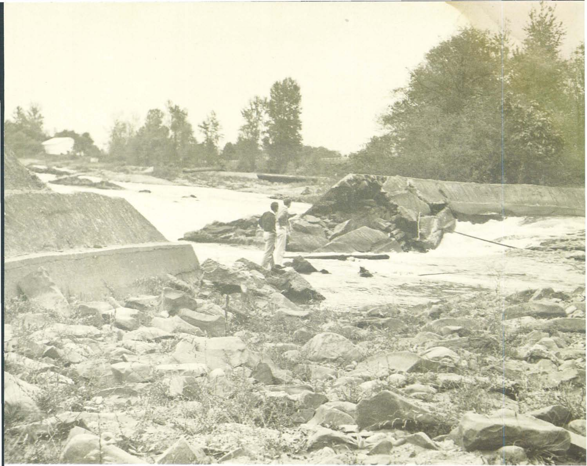
Broken dikes - foreground rocks are tillrace bottom
