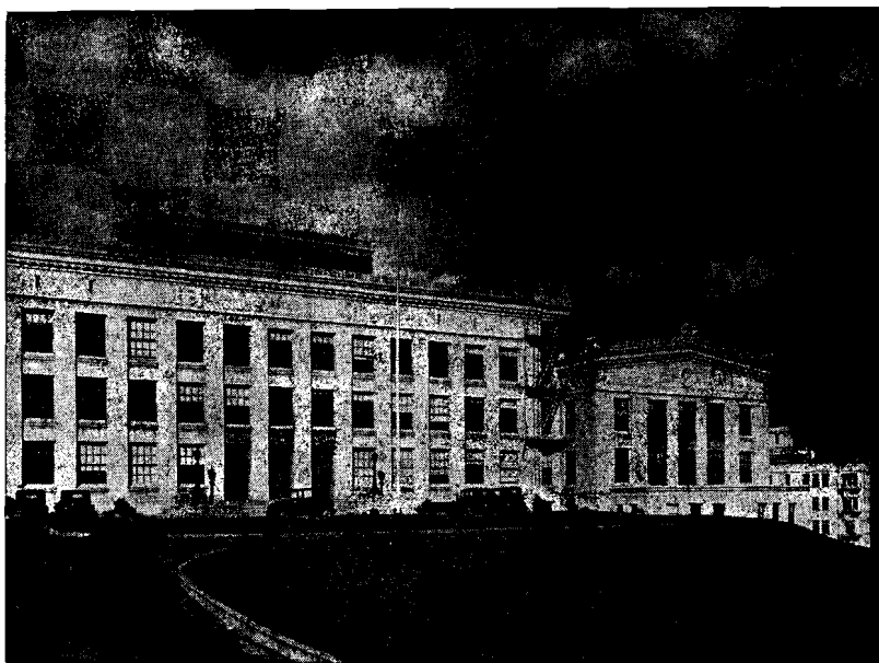
Below: Medical School Building.
