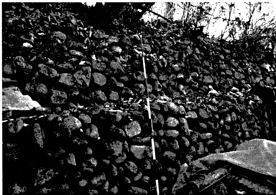
Figure 90. The stone mound tomb in Sinmae-ri (A close look and its part modified as a wall).
