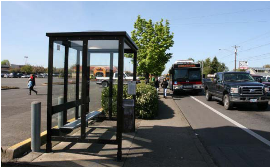
Figure 37: Current bus stop.
