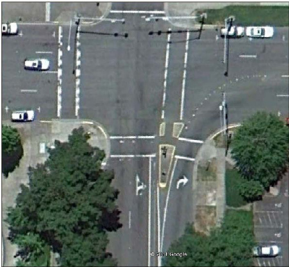
Figure 41: Intersection of Summer Street and Marion Streets.
