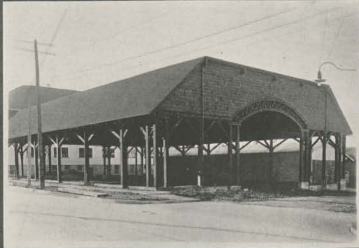
The Drill Shed
