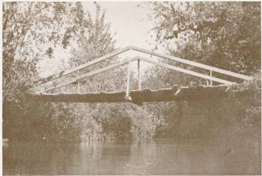
THE MILL RACE BRIDGE
