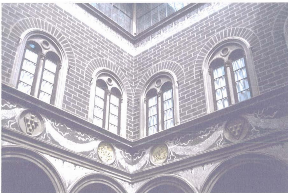
Figure 10. Michelozzo di Bartolomeo, Palazzo Medici courtyard : roundels with mythological scenes and arms of the Medici, begun 1444. Florence, Italy.
