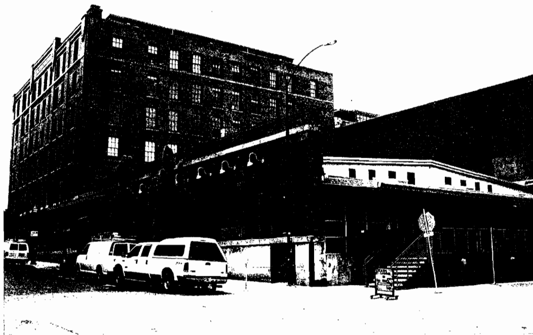
Figure 12: Southeast view of Crane Company Building. Single-story restaurant space is currently under renovation (photo by author, 2010).
