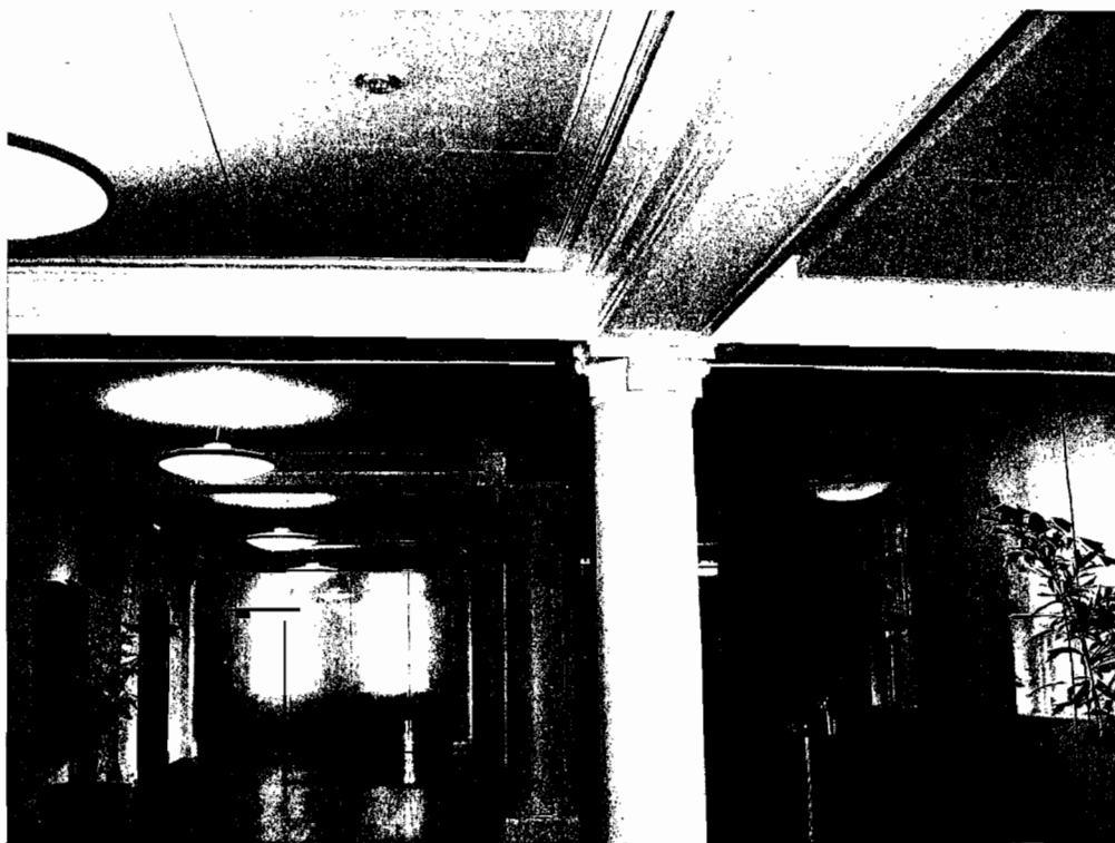
Figure 15: Second Floor space was given a high finish to serve the historic Crane Company offices and is now occupied by Guardian Management Company. (Photo by author, 2010).
