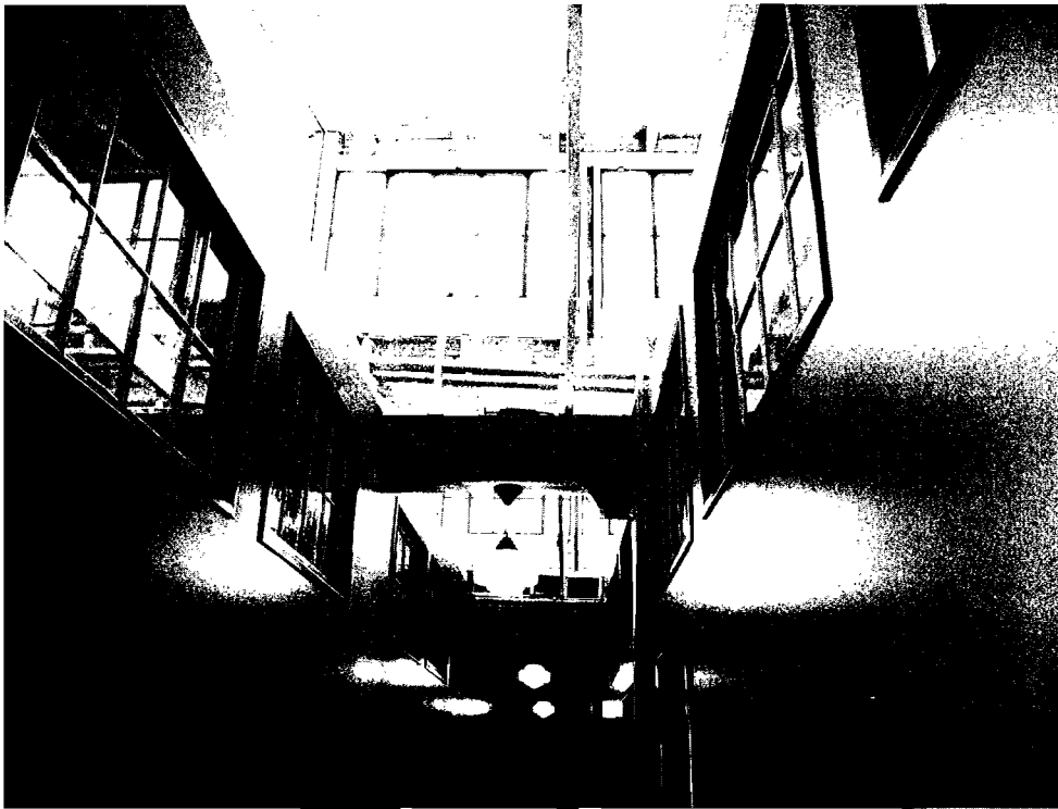
Figure 22: Northwest Fence & Wire Works Building deteriorated exterior wood windows were repurposed in upper floor hallway to maximize the visibility of and day lighting from the historic saw-tooth light monitor above (photo by author, 2010).
