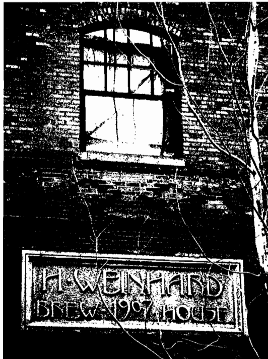
Figure 4: Historic sign identifies place as H. Weinhard Brew House. It includes the 1907 construction date. A historic window is centered above. (Photo taken by author, 2010).
