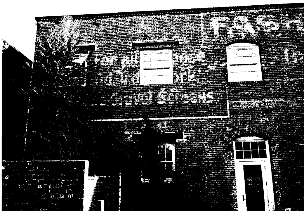
Figure 19: Northwest Fence & Wire Works Building north elevation has evidence of ghost signage from both Fashion Stables and Fence company occupancies (photo by author, 2010).
