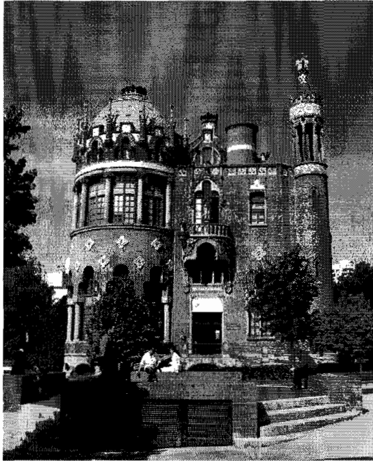
Figure 4.3 Pavilion of the Hospital de Sant Pau (M. Landers 2009)
