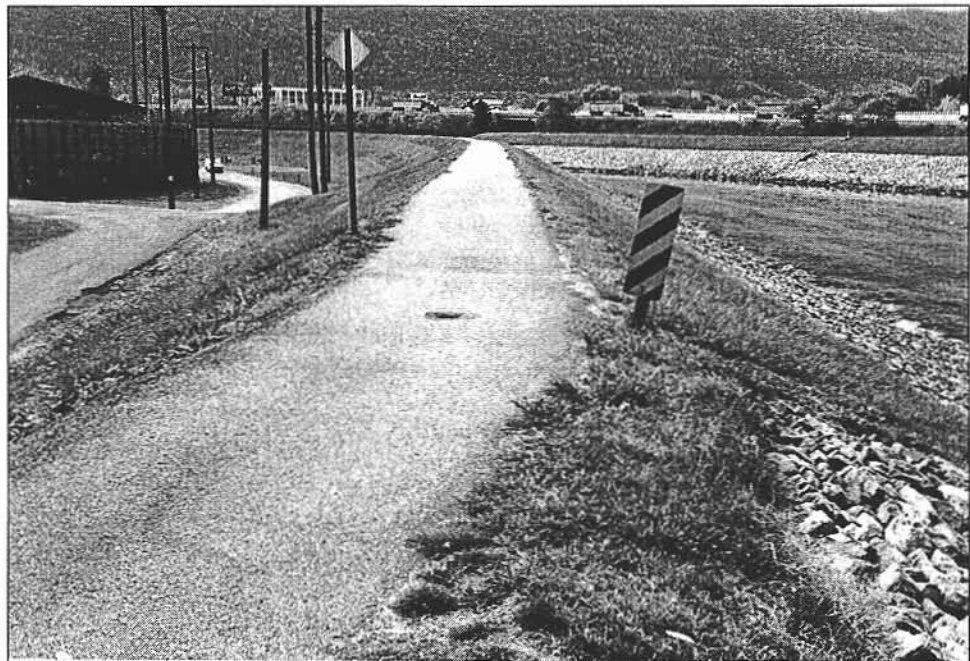
Asphalt, multi-use trail on flood control levee in Williamsport, Pennsylvania.
