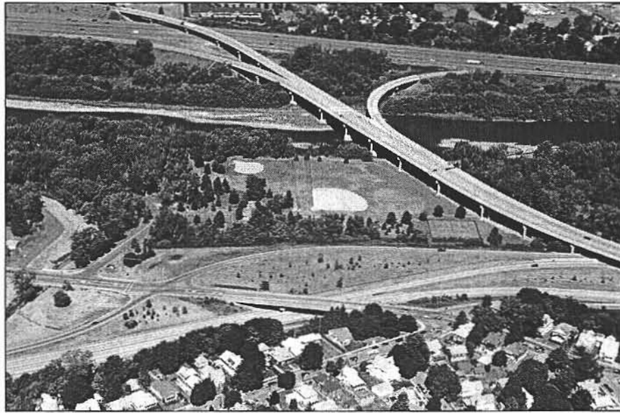
View of Port Dickinson Park, I-88 bridge, Chenango River and, across the river, the proposed site of the Otsiningo Park Trail Extension.
