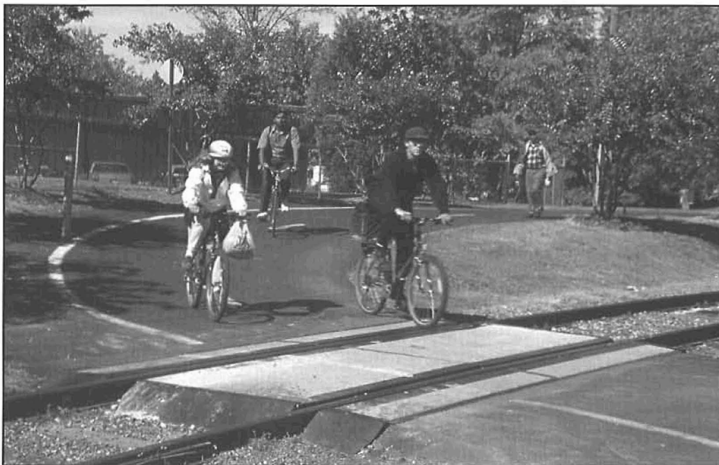
A multiuse path along an active rail line creates an important transportation link
