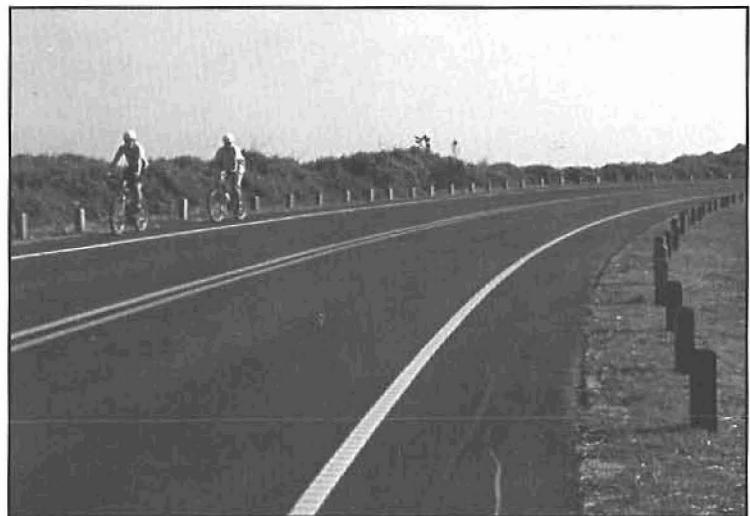
Wide paved shoulders provide safer conditions for motorists and bicyclists
