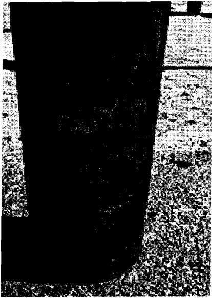
Avoid Bollards. How did these gouges (above and below) get here? Most likely each scar created scars on the rider. Use signing, tight corners and medians to keep autos out (They don't want to be there anyway). Design them so that emergency vehicles can go over the curbing or over the top.
