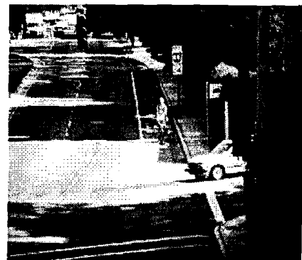
Below: Gainesville's 13th Street & Archer Road high speed turn lane was seen as too complex to cross by novice riders. Many bicyclists rode against traffic on the far side, creating serious conflicts at this blind intersection. Special bike lanes were added (bottom photo) to assist the merge.
