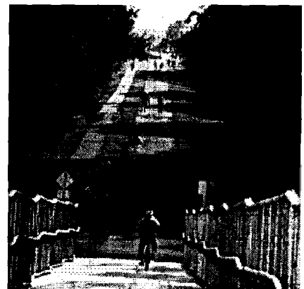
Pinellas Trail -- 12 feet + 6 foot pedestrian trail. Pedestrians use separate trail when wheeled use is heavy. Other times they mix by choice.
