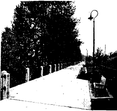
River fronts offer one of the few occasions where sidewalks can transport bicyclists with minimal conflict with motorized traffic. Sufficient width must be provided to reduce conflict with pedestrians.
