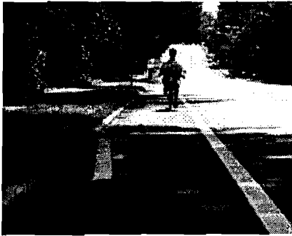
When older drainage facilities extend into the paved area, mark the hazard to steer bicyclists around them. New construction on state roadways uses inlet style drainage, which keeps lanes free of these hazards.
