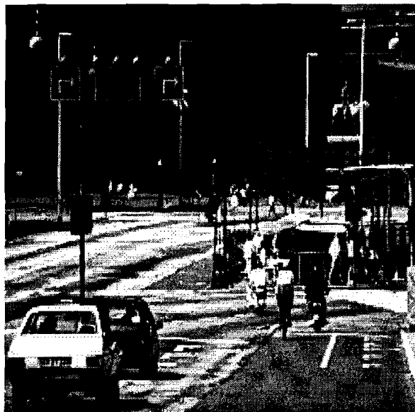
This specially marked lane in Copenhagen, Denmark illustrates a method used when bicycle and motorist volumes are high. The bicyclists and motorists each have their own signal for right turns and through movements.
