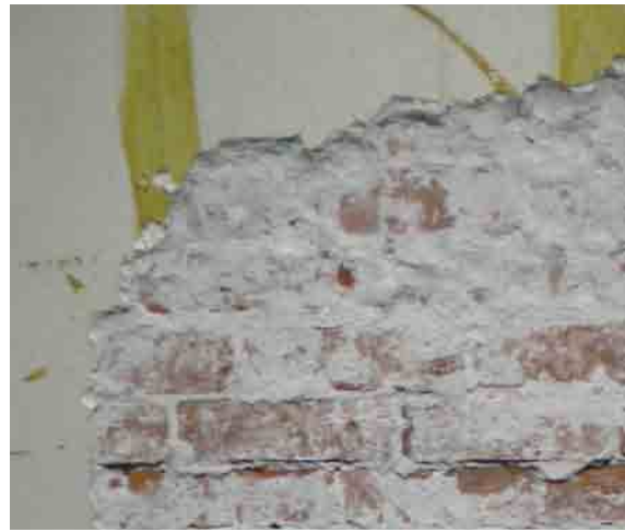
a) brick wall with plaster
