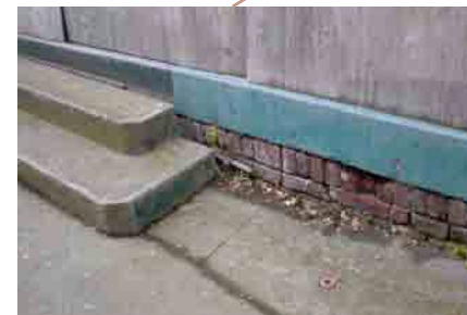
i) brick structure supporting concrete slab
