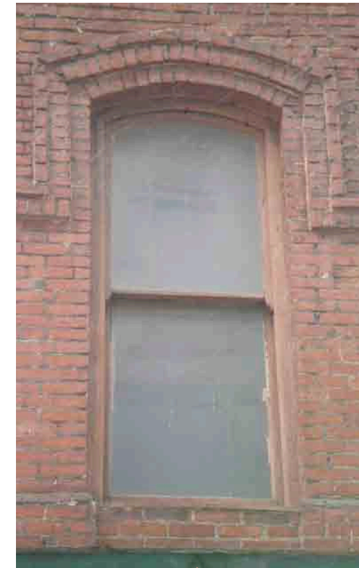
e) typical exterior window of hotel room
