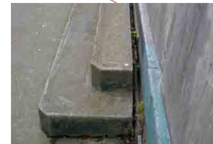
j) concrete steps leading to storefront
