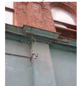
m) stucco finished brick pilaster
