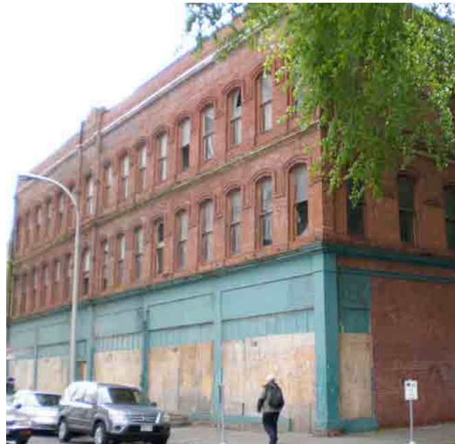
a) view from NW of storefront
