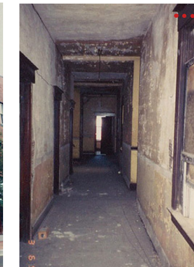
3rd floor pre-renovation
