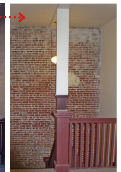
Stairwell brick wall exposed
